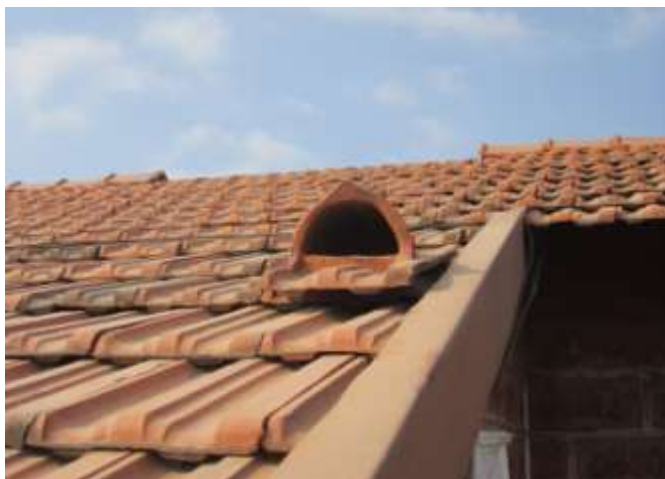
Traditional mangalore tile roofing with stag vent tile.
