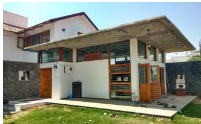
Modern concrete roofing and traditional sloped mud tile roofing
